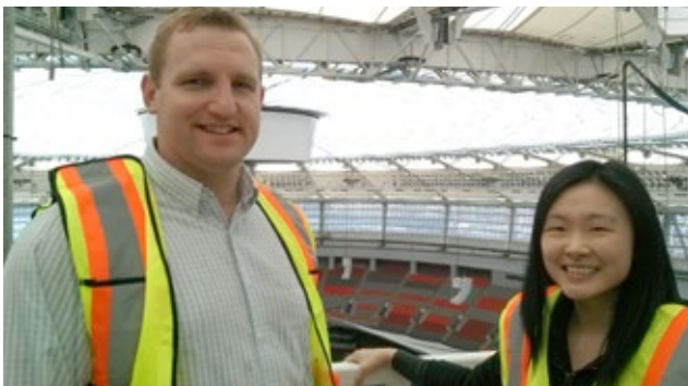
Auditors Evan Machin and Shannon Chang examine BC Place's drainage system as part of their audit work.
