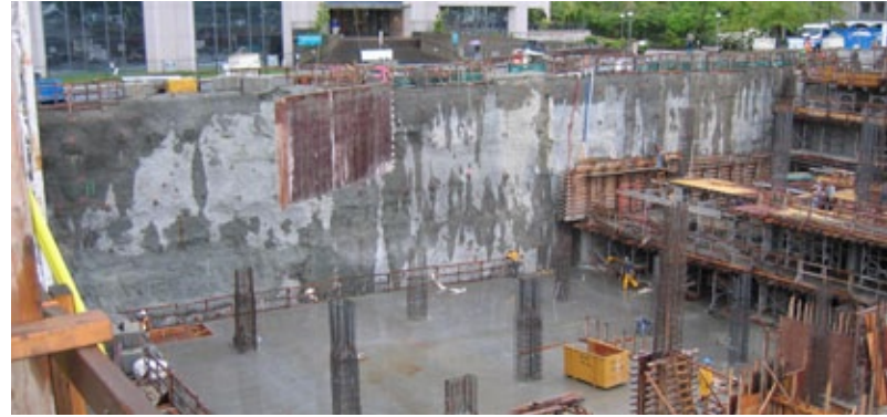
Early construction on the facility
