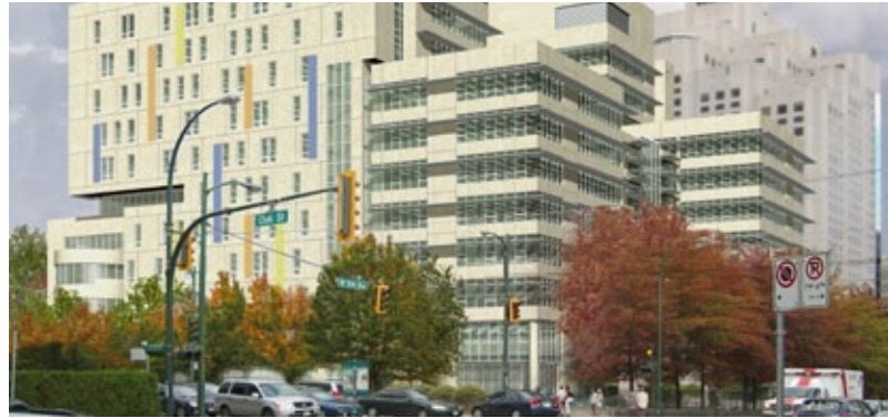
Distant view of the completed Academic Ambulatory Care Centre, part of the Vancouver General Hospital
