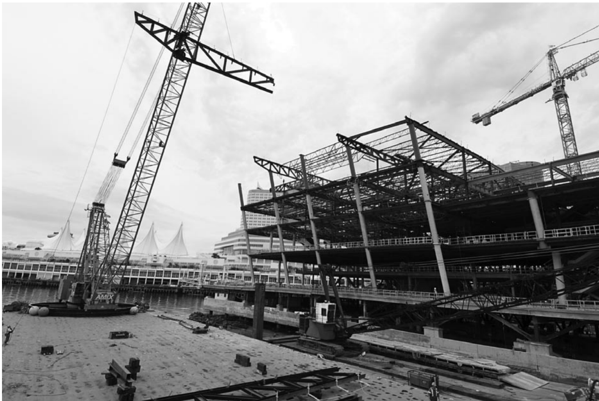
Steel fabrication at the site
