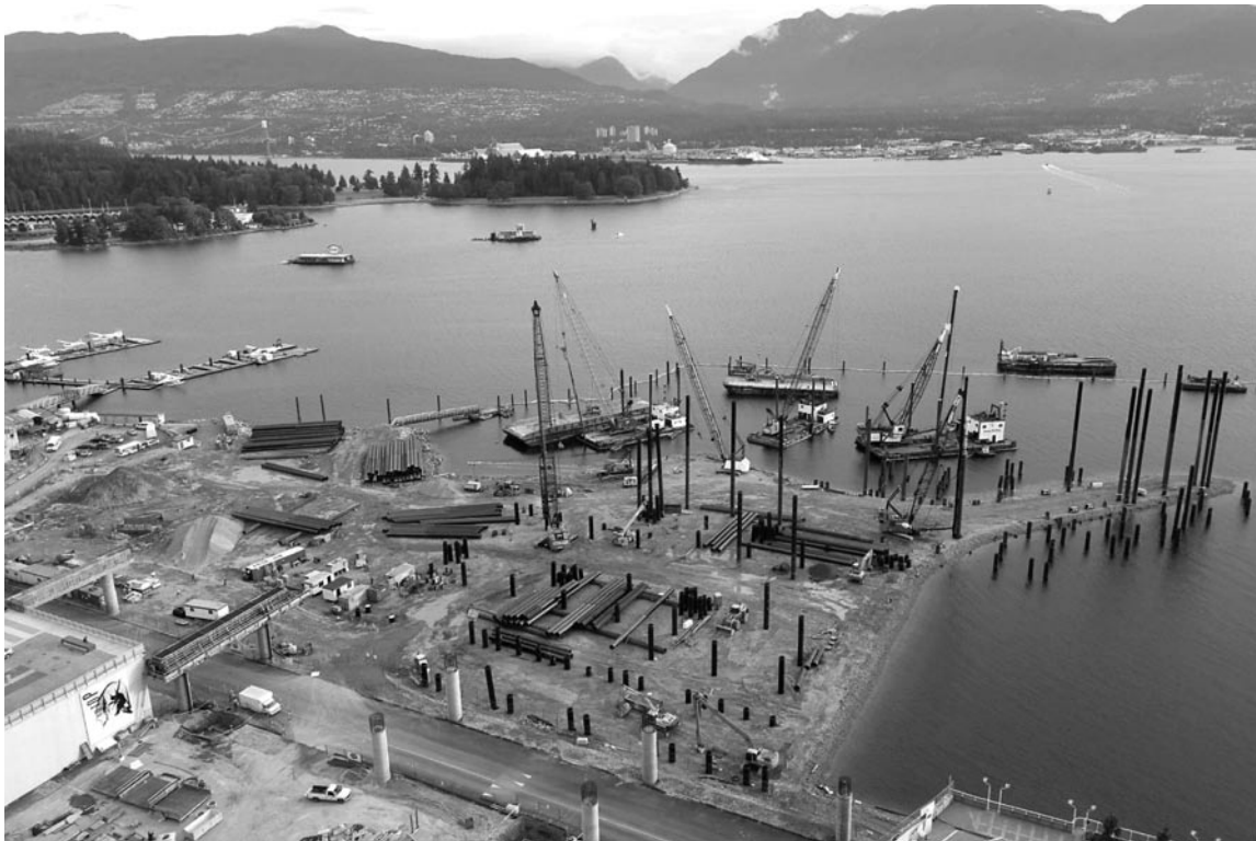
Construction site in June 2005
