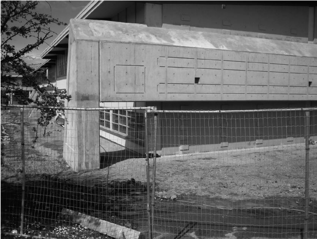
Seismic Upgrade of Mount Douglas Secondary, Greater Victoria School District
