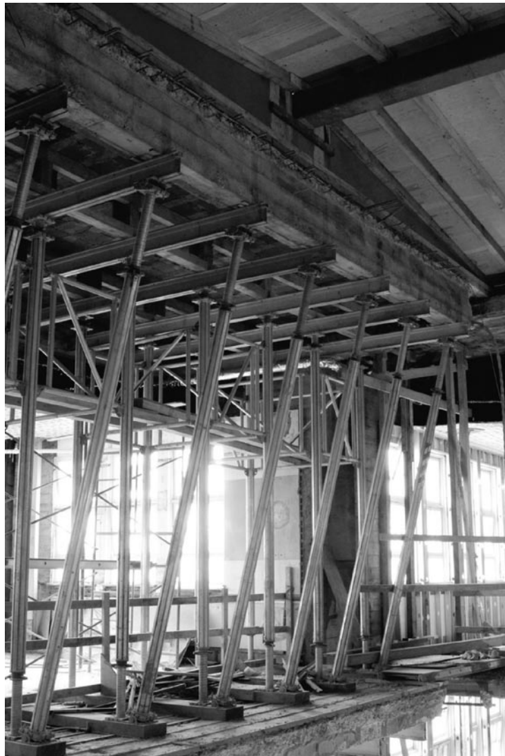
Seismic Upgrade of Vancouver Technical, Vancouver School District
