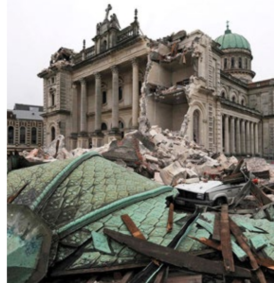
Debris crushed a car outside the Christchurch Catholic Cathedral after a 6.3-magnitude earthquake hit Christchurch, New Zealand, Feb. 22, 2011.
