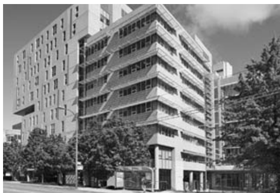
The Gordon and Leslie Diamond Health Care Centre is an example of a government capital project carried out under a P3 procurement and financing model. Source: PSPBC website
