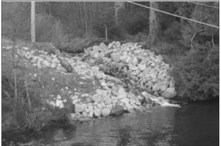
A stream bank stabilization project on a tributary of the Salmon River
