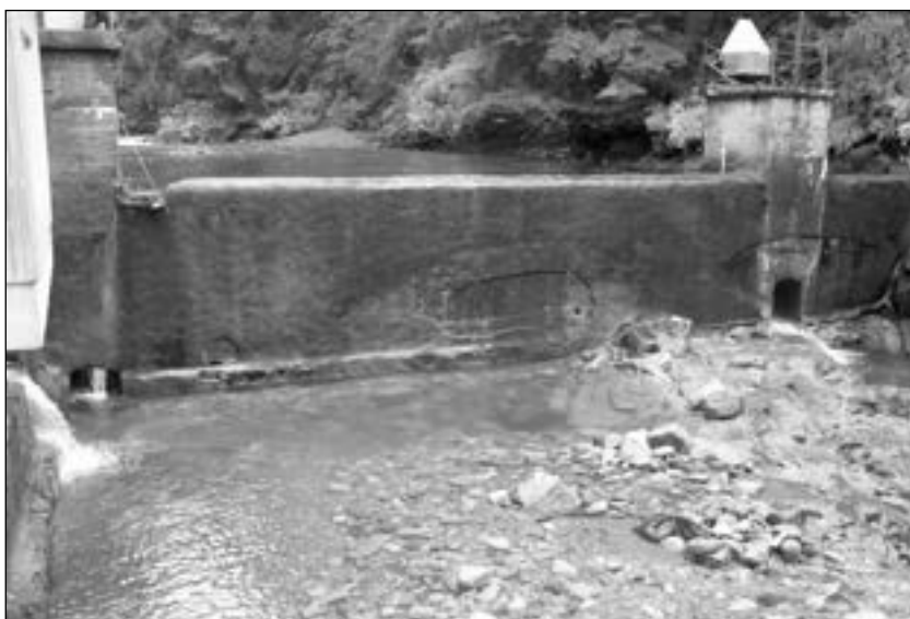
Water impoundment obstructing fish passage
