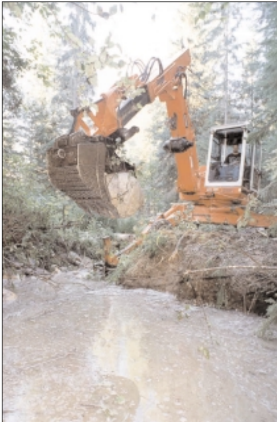
Mechanical spider performing work in creek as part of a Forest Renewal BC-funded project to restore fish habitat
