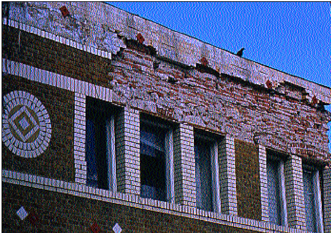
Damage to building masonry
